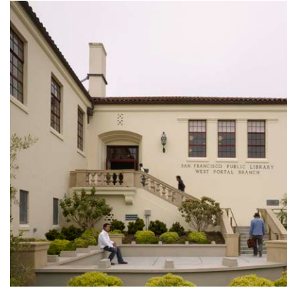
WEST PORTAL LIBRARY
