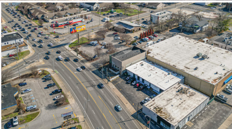
SITE AREAL (LOOKING WEST)
