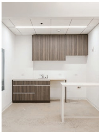
Renovated Office Space
