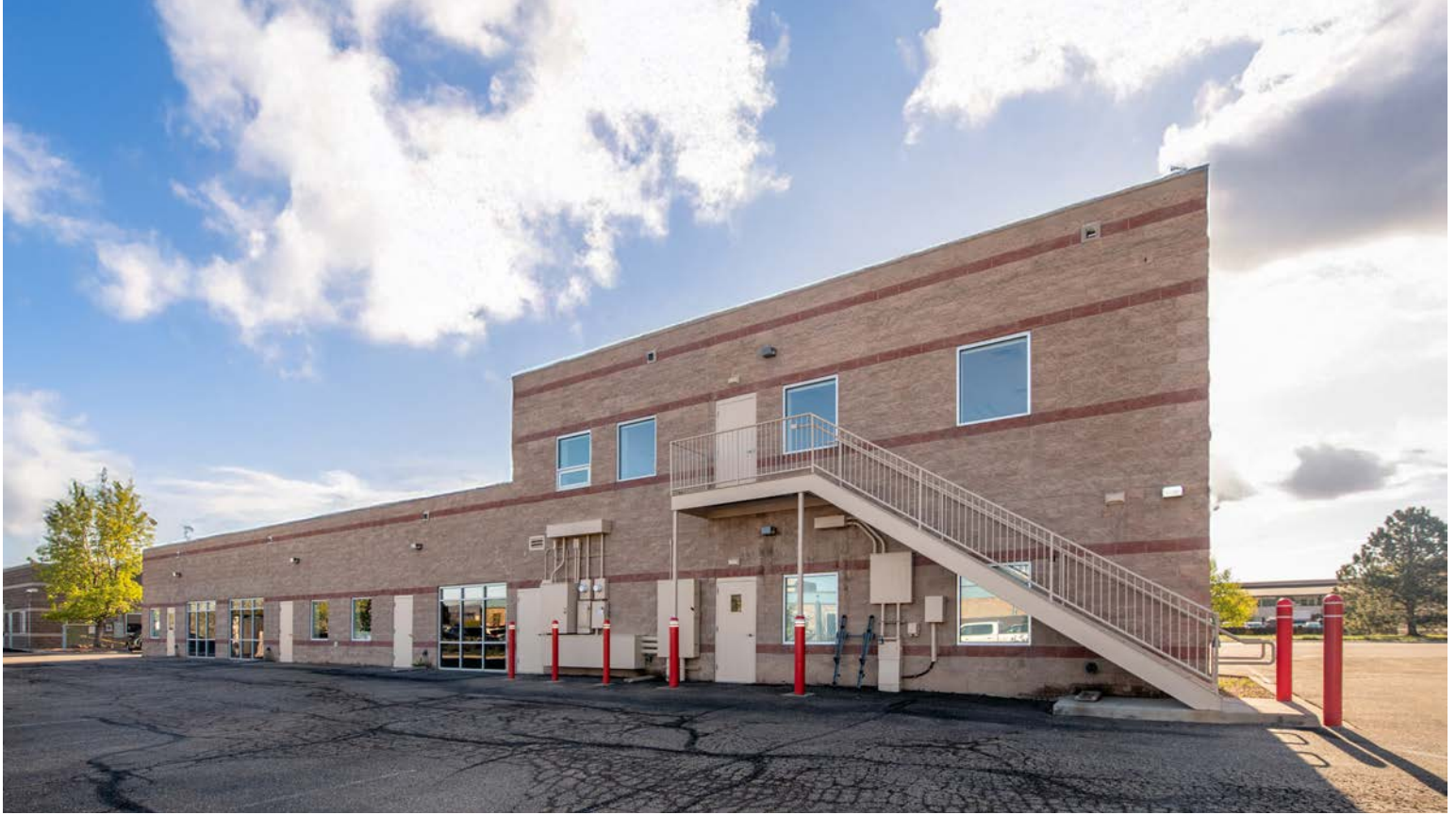
West Elevation from SW Corner
