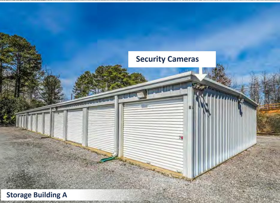
Storage Building A
