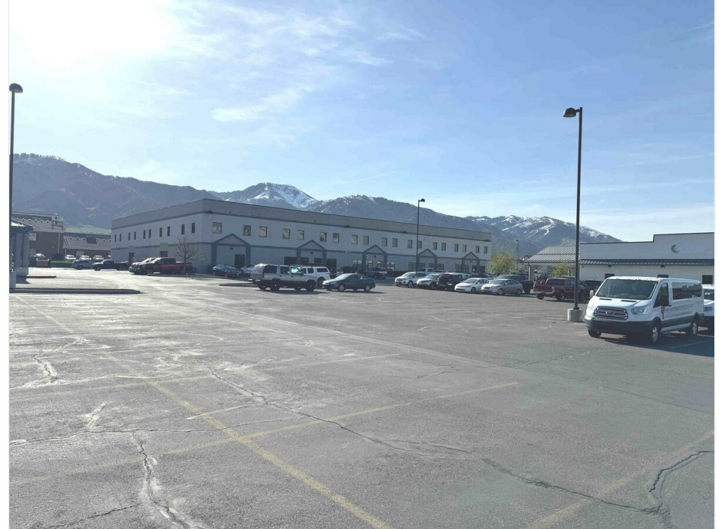
Parking Lot view
