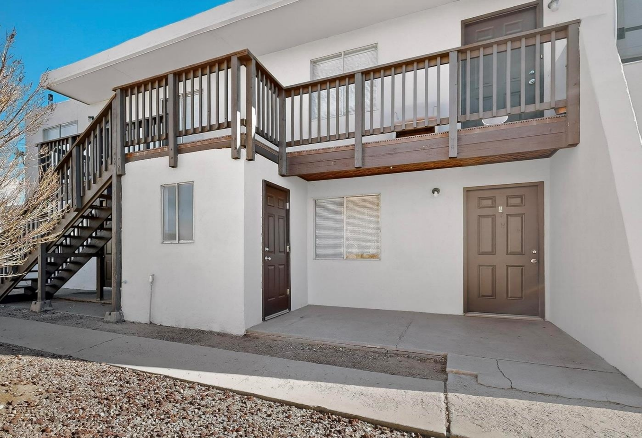
Front of Building
